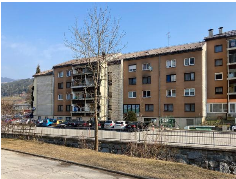
Slika 8 Fotografija stavbe pred prenovo (Vir: https://infinitebuildingrenovation.eu/cases/infinite-case-study-slovenia )
